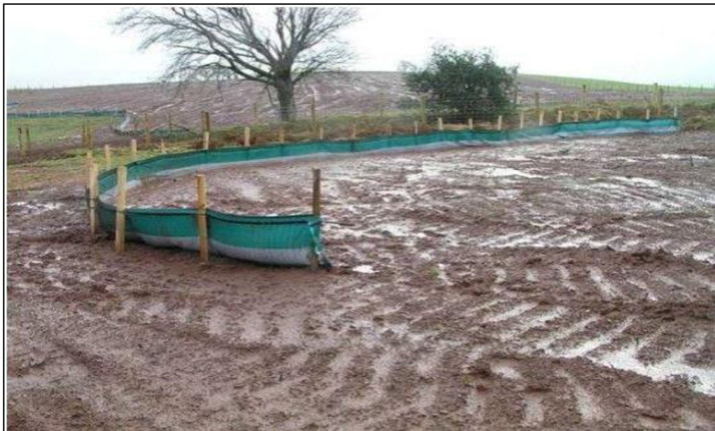
Figure 3.2b – Typical Silt Fence Image
