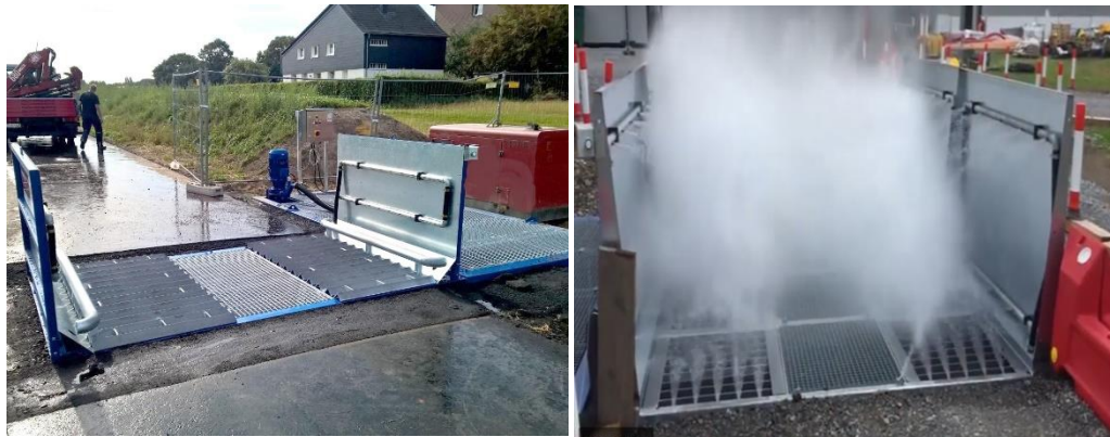
Figure 3.2e Example of static wheel wash systems
